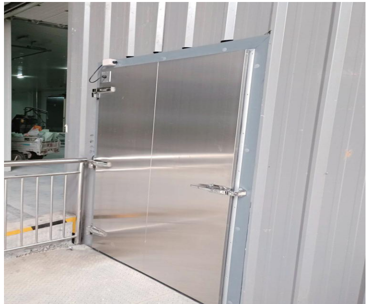
Cold Storage Doors
